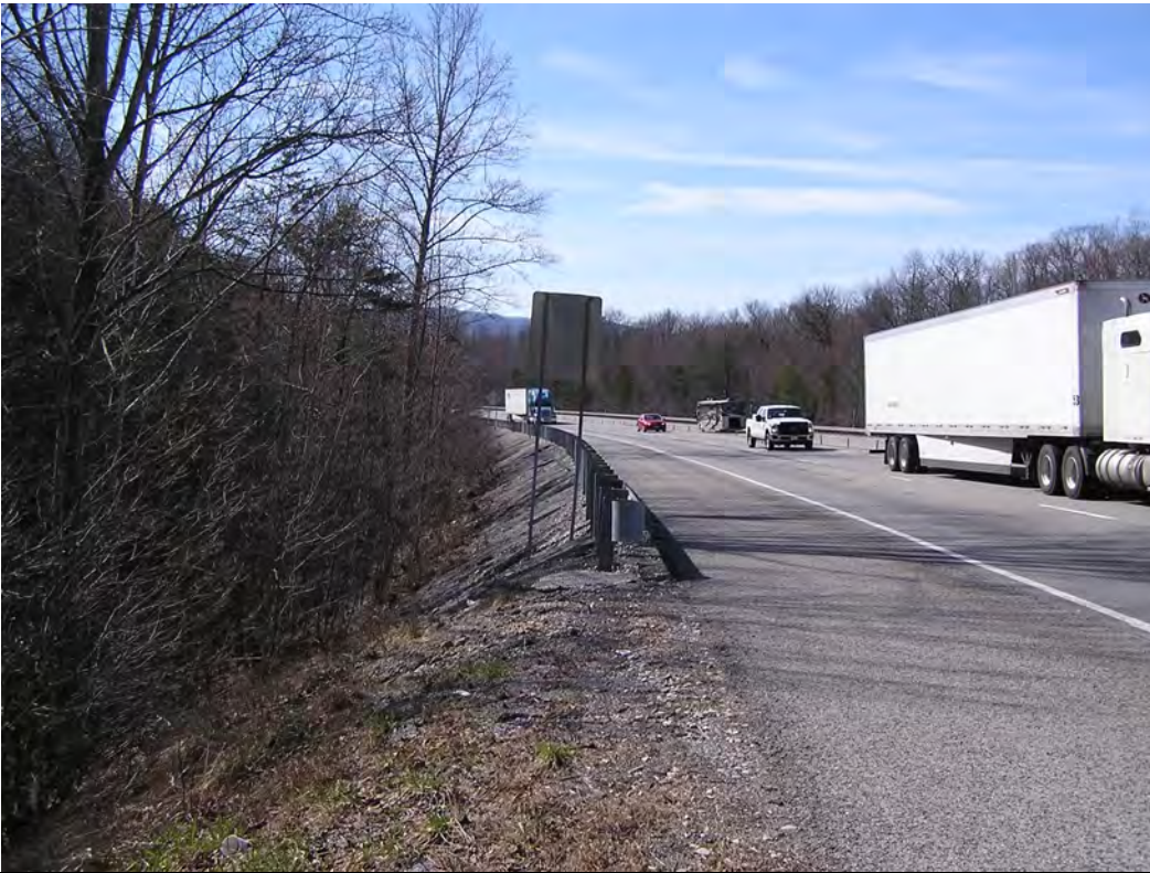
Photo 3: STA 166+00 RT. View of I-75 northbound lanes above STR-2 facing south.
