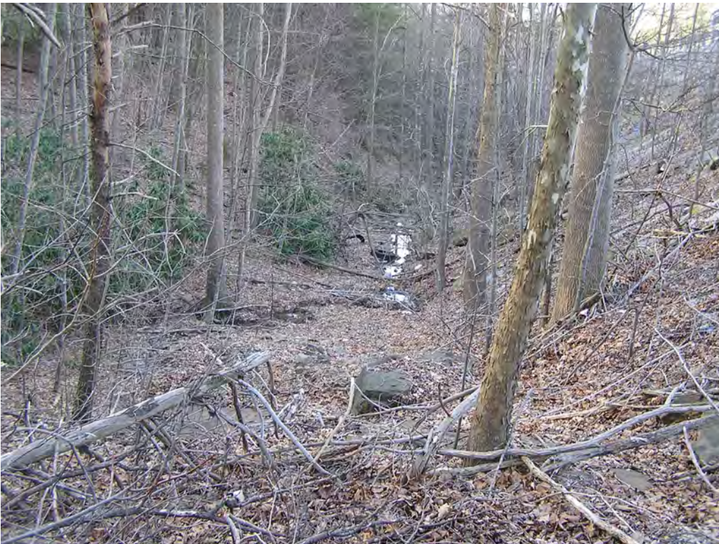
Photo 4. STA 166+00 RT. View of STR-2 facing south (downstream).
