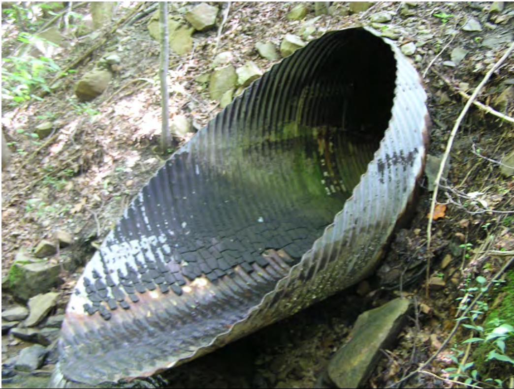
Photo 1: STA 153+50 RT. View of STR-1 (Big Branch) facing southwest.
