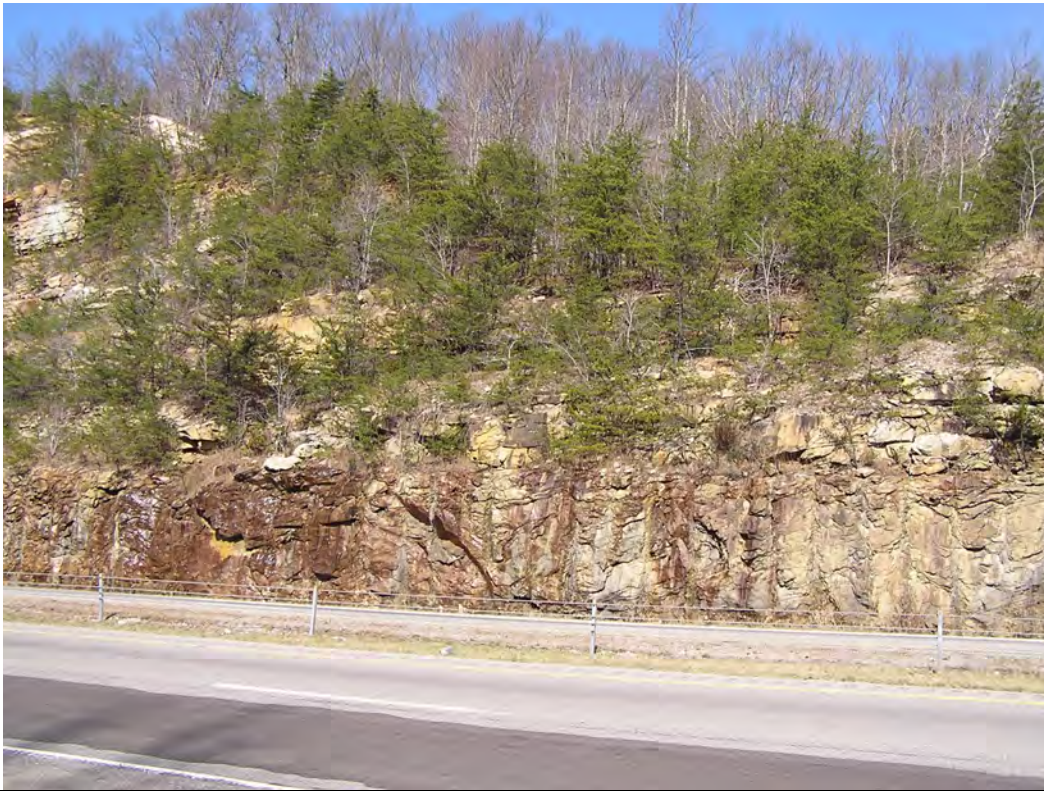
Photo 5: STA 190+10 RT. View across I-75 from STR- 3 facing northwest.
