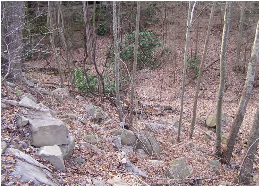
Photo 8. STA 209+75 RT. View of STR-4 facing southeast (downstream).
