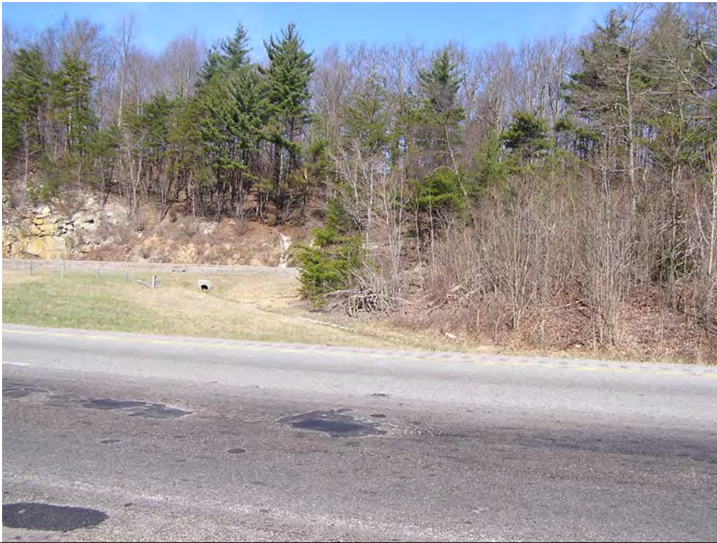
Photo 7: STA 209+75 RT. View facing northwest.
